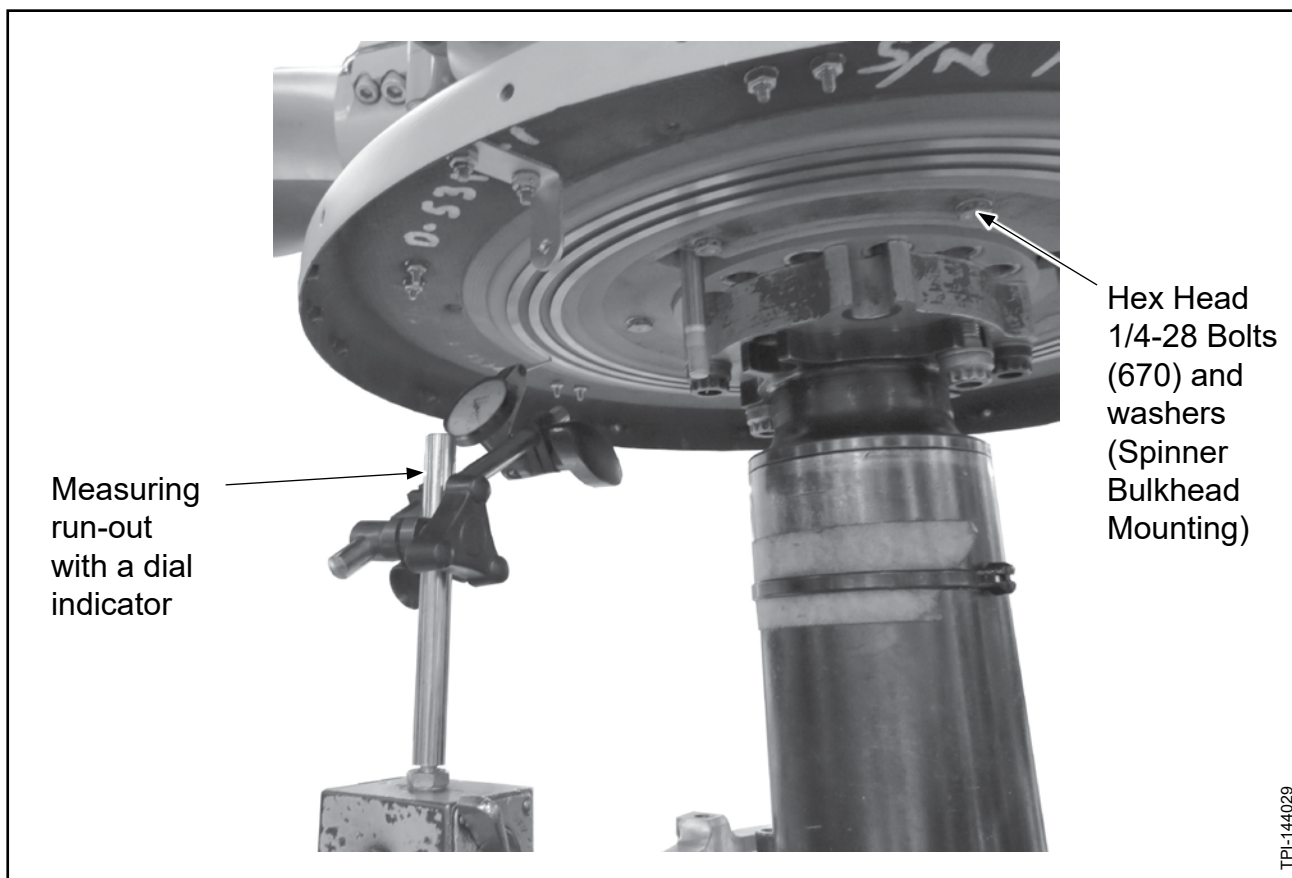
Installing the Spinner Bulkhead Figure 7-27
